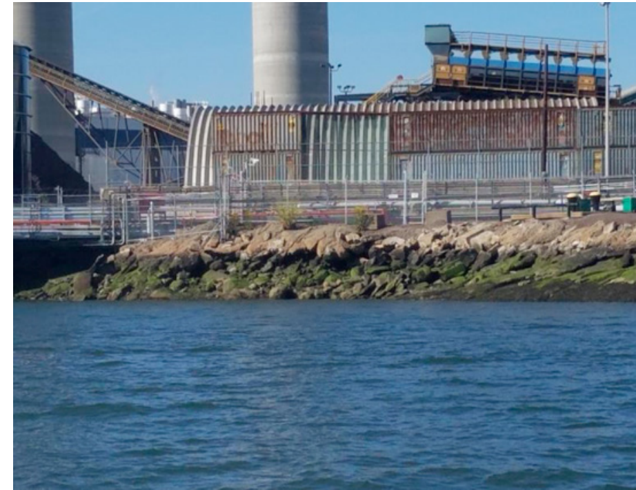
Figure 9: Riprap located at Prolerized
