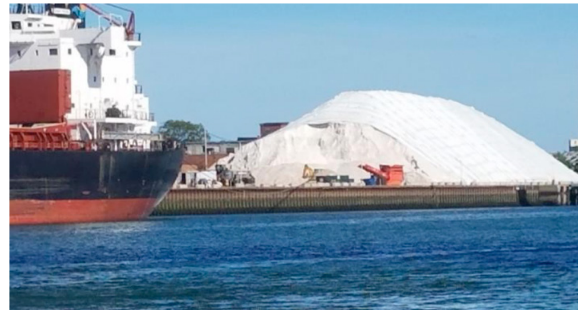
Figure 10: Bulkhead located at Eastern Salt
