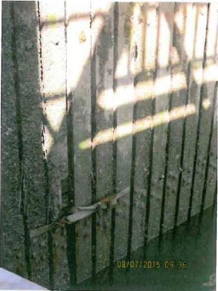
Damage to wave fence, held together with ratchet straps
