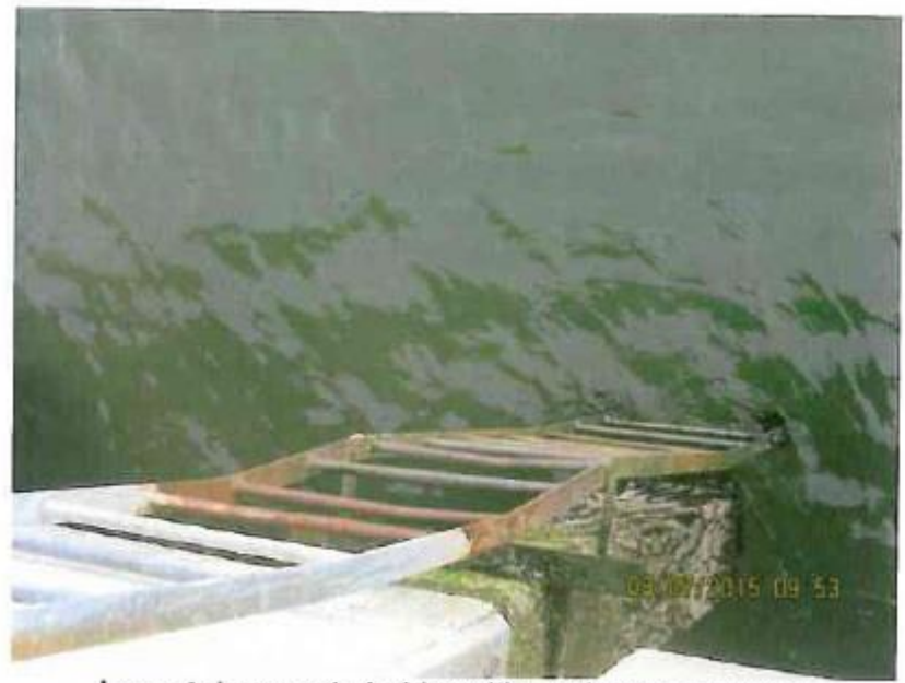
Impact damage to ladder with moderate corrosion
