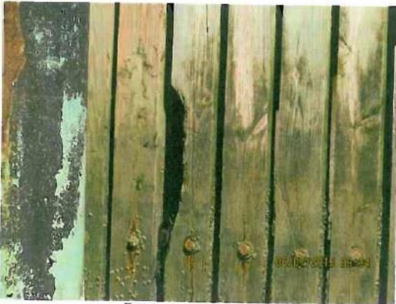
Damage to wave fence
