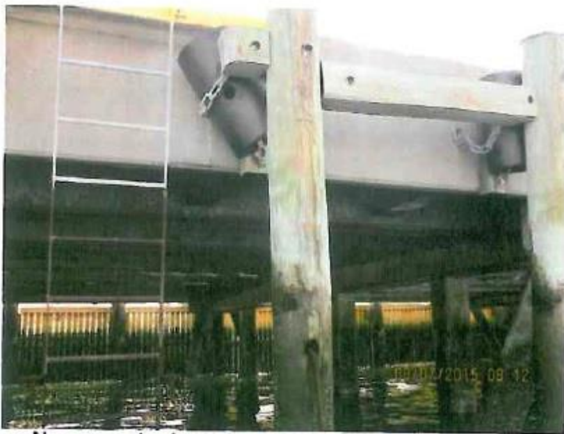
Neoprene circular pad connection failure due to scaling concrete
